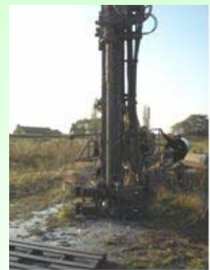
Water Flush Drilling
